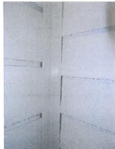
Internal corner horizontal cladding
